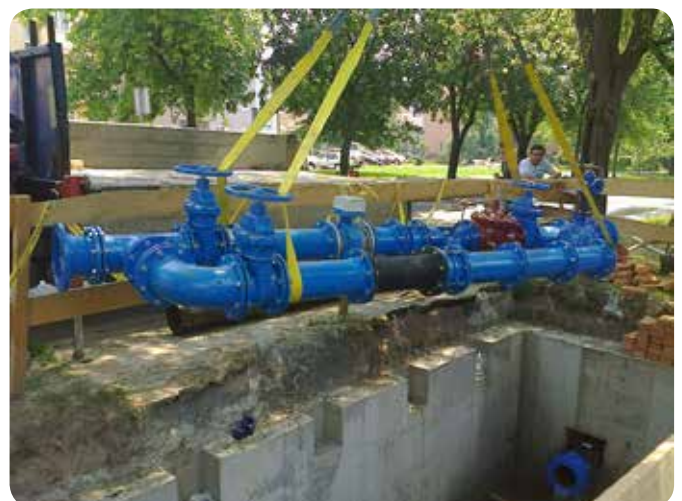
An example of the installation of already combined instrumentation and control equipment inside the inlet chamber with a crane.
