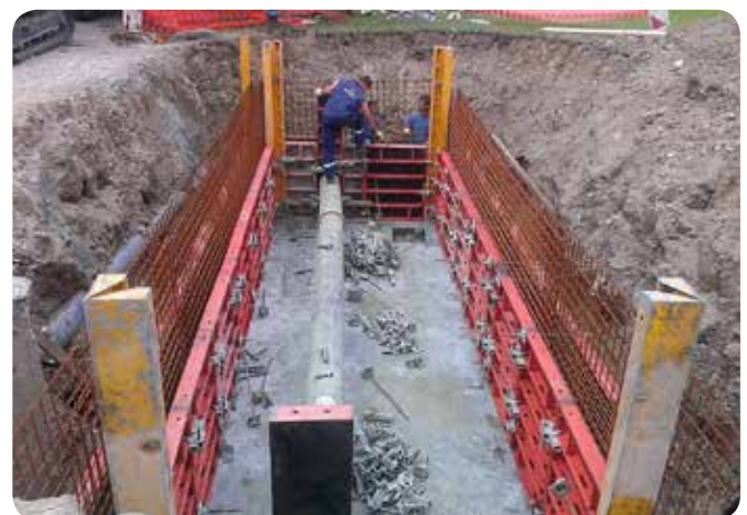
An example of a chamber during construction. Ready-made industrial metal formwork is used for concreting.
